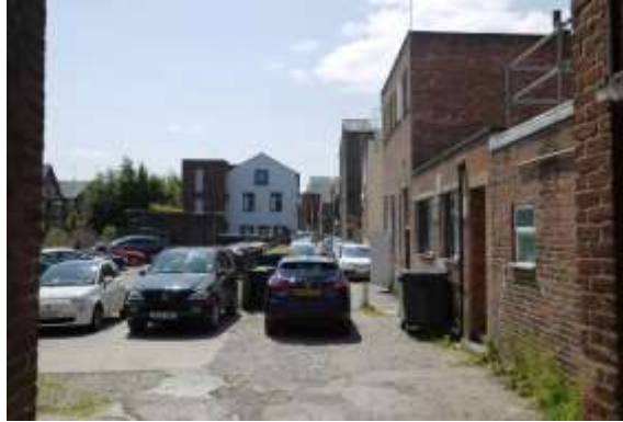
Mixed road surfaces along Back Grafton Street could be enhanced and parking restricted to create an attractive pedestrian thoroughfare
