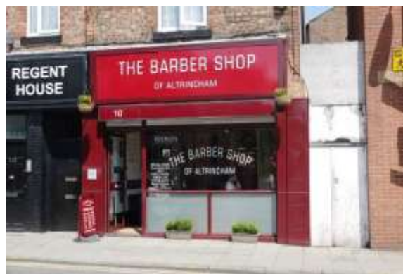
Example of a traditional shop front at 10 Regent Road. However the fascia is quite large.
