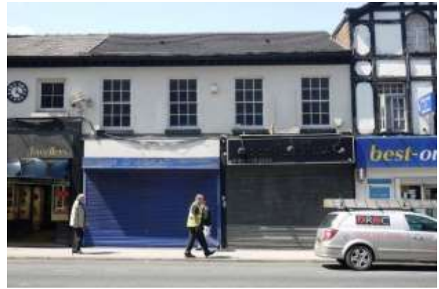
24-30 Railway Street are three properties that have been extensively altered and have potential for enhancement. Note the inappropriate (and vacant) shop fronts with roller shutters and recently painted façade. Traditional windows survive on 24-26 but have been replaced with uPVC in an inappropriate square design at 30.
