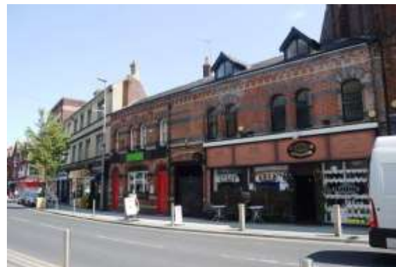
Two shop fronts exhibiting signage that is too bright or overly large and repetitive. Note the proliferation of A-boards on the street
