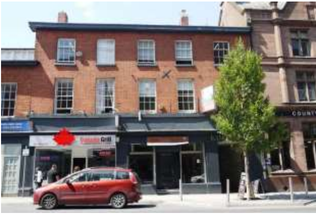
A good example of a building (36-40 Railway Street) that retains its original windows and is in use across all three floors.
