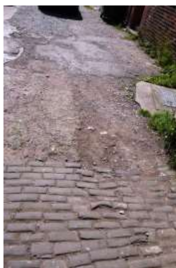
Traditional paving on Back Grafton Street
