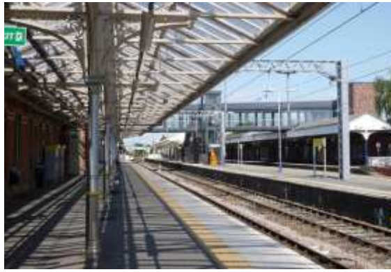
Railway station platform buildings
