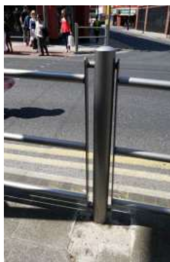
Modern barrier systems
